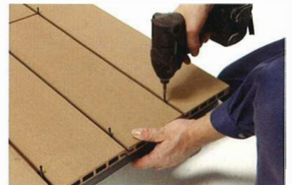
11. fixing Side boards
