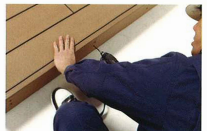
11. fixing Side boards
